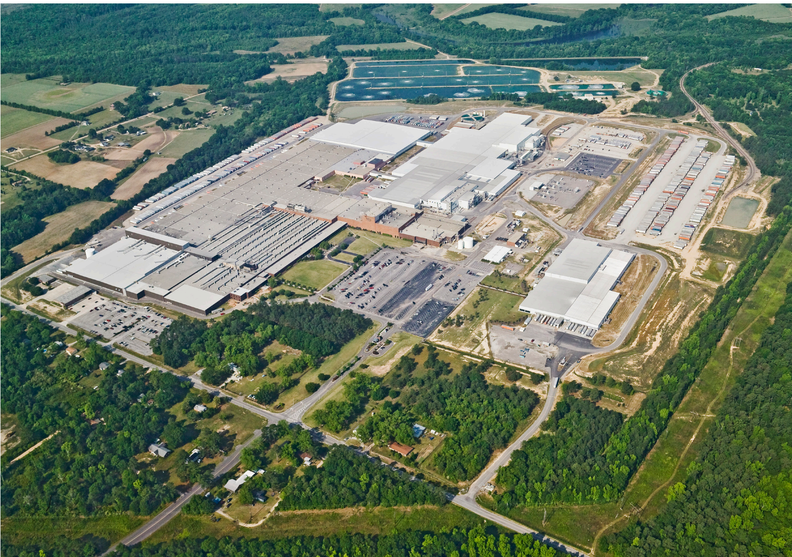
Large-scale manufacturing facility in South Carolina
