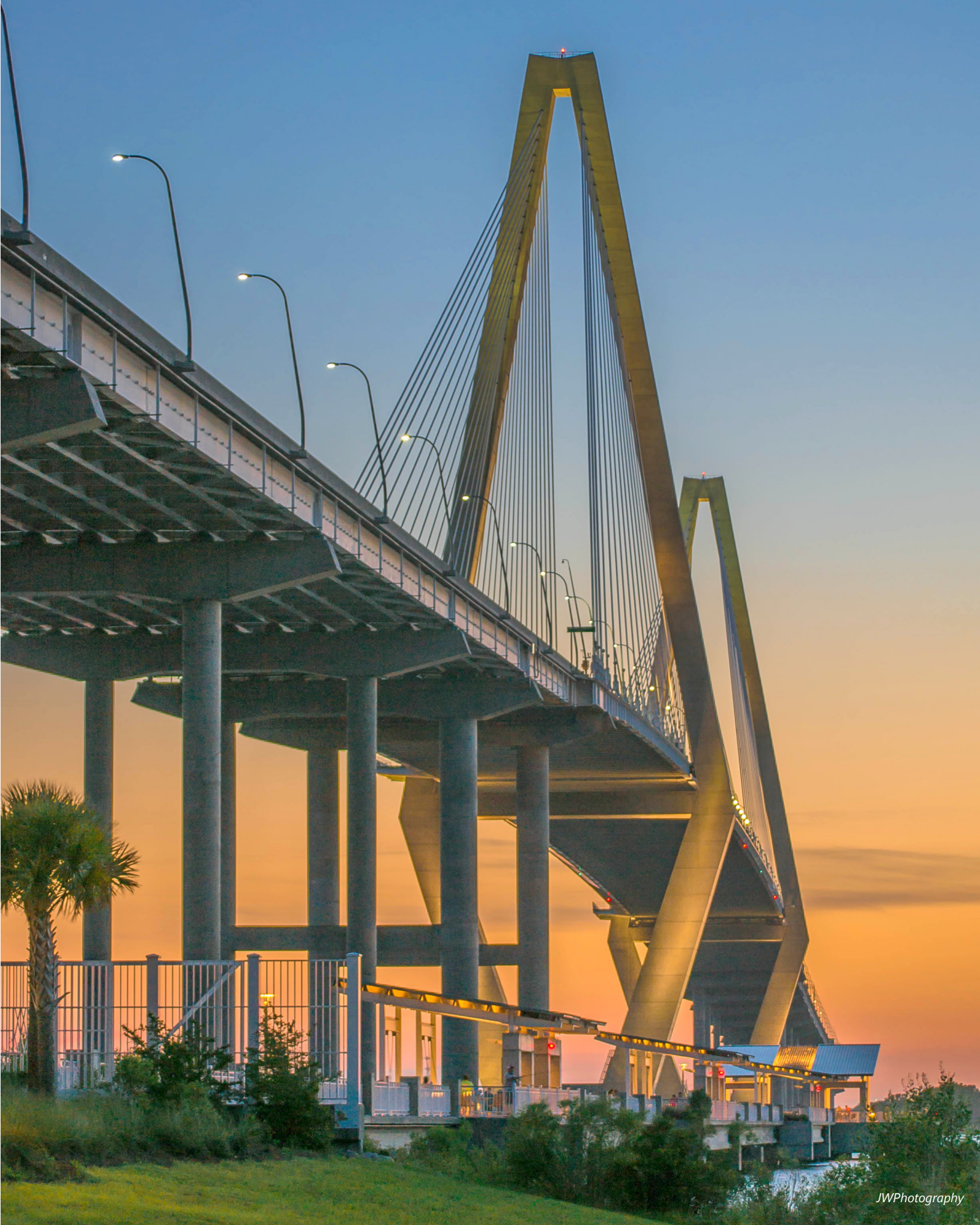
The Arthur Ravenel Jr. Bridge, a cable-stayed bridge over the Cooper River in Charleston, SC
