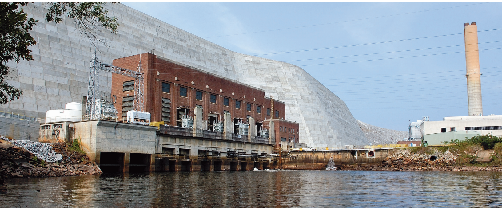
Located at the base of the Lake Murray Dam, SCE&G's 250 MW McMeekin Station uses cooling water drawn from the bottom of the lake, thus increasing the plant's efficiency and reducing air pollution.
