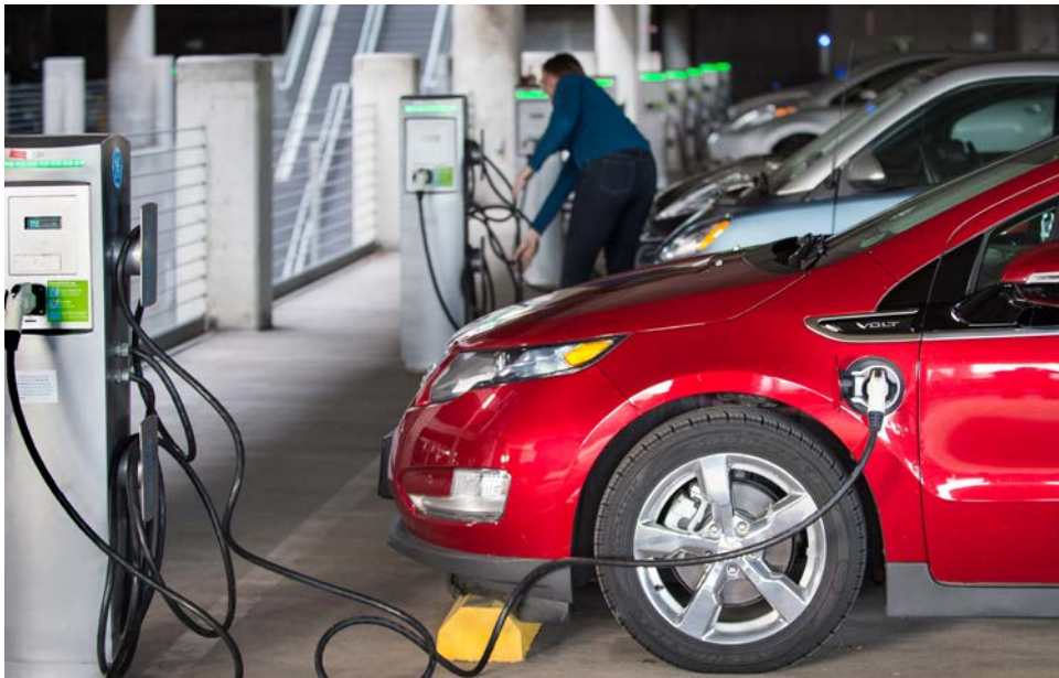
Public charging stations typically have one or more “Level 2” charging units. Photo by Dennis Schroeder, NREL 35149
